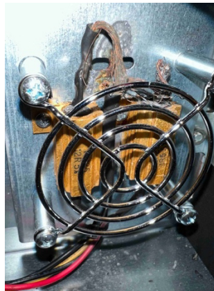
Figure 1: Example of overheated and frayed expansion chassis load wires.
